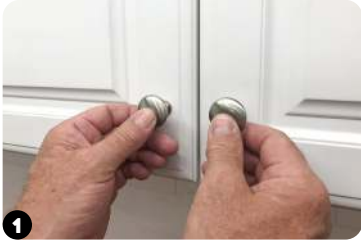
1 Place hardware (measure as needed) to find position you like; mark hole location
