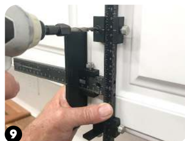
9 Drill through Drill Guide for top hole.
