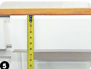
5 Measure height of drawer front.
