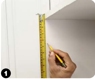
1 Mark center of hinge plate.
