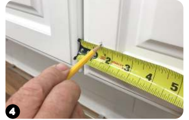
4 Measure from side of door to mark.
