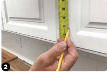
2 Measure from bottom of door to mark.
