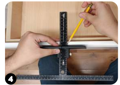
4 Use half of measurement from Step 3 to mark center on top of drawer.
