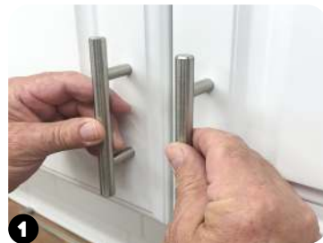
1 Place hardware (measure as needed) to find position you like; mark bottom hole location.
