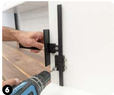
6 Flip tool to bottom of cabinet, position tool with Large Stop and T-Square firmly against cabinet surface, and drill second set of holes.
