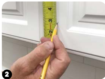
2 Measure from bottom of door to mark.
